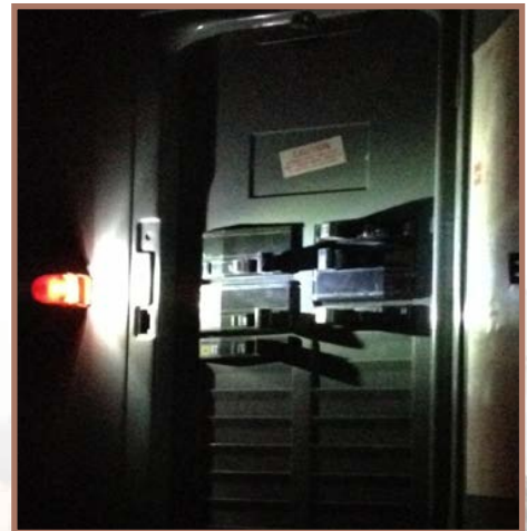
and Fuse Box
